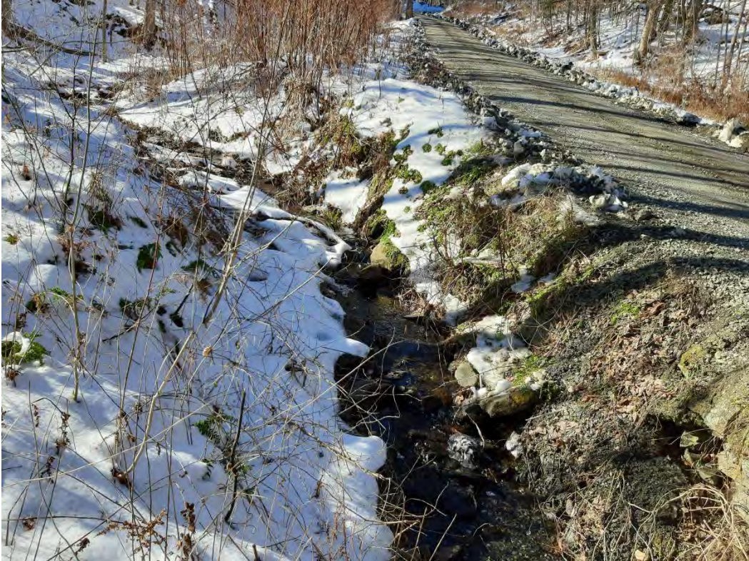
Culvert 21 inlet view of upstream
