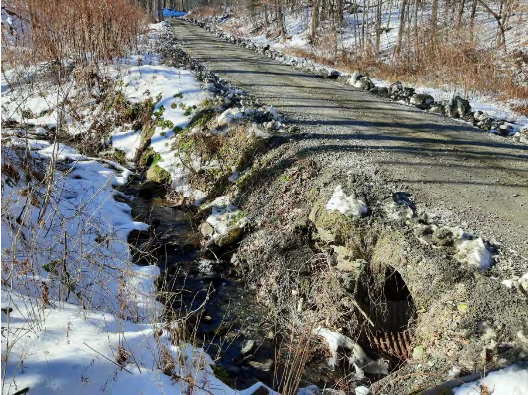
Segment 31797 – Culvert 21 inlet of an existing 48" x 48" x 20ft metal culvert
